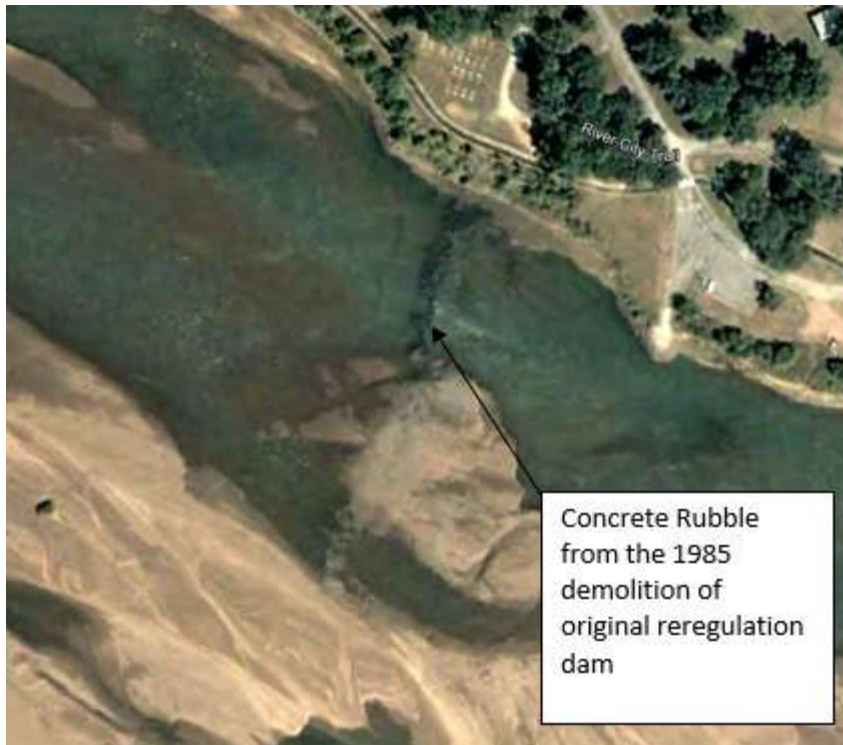
Figure K-2: Aerial photo showing rubble within the channel from reregulation dam demolition
